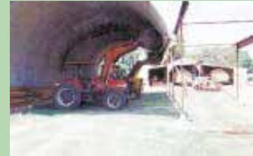
One side bolts to a 4-ft. high wood wall and the other side to a 10-ft. high steel frame.
