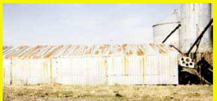
Note how Vaessen used pie-shaped panels to make the roof.
