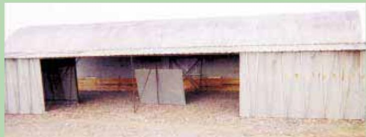
Miller used some of the pie-shaped roof panels to make partial walls along the open side of the building.
