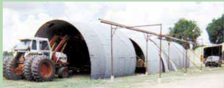
The half-bin sections were hauled by a loader tractor to a site prepared for the shed
