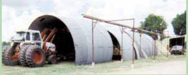
The half-bin sections were hauled by a loader tractor to a site prepared for the shed
