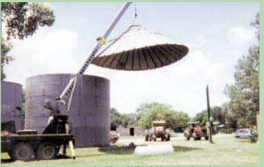
Truck-mounted crane was used to lift roof off each bin and set it on the ground.
