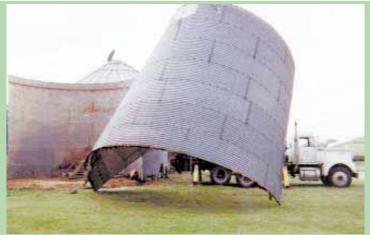
After bin was cut vertically down each side, a crane was used to lay each half down.
