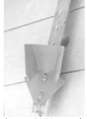
As soon as post starts to move up, wings on the top half of the anchor flatten out to keep post from going up any farther.
