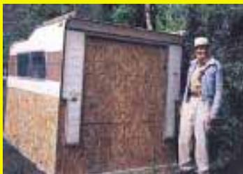
one of my ideas. It's a way to make use of an old pickup topper. I used it as a roof for a tool shed that stands in the back yard. The sides are made from particle board. I put a hinged door in the wood on one end. Many of the old toppers don't fit newer trucks so there are a lot of them around. **(Bill Miller, Box 151, Landis, Sask. S2K 2K0 Canada)**
