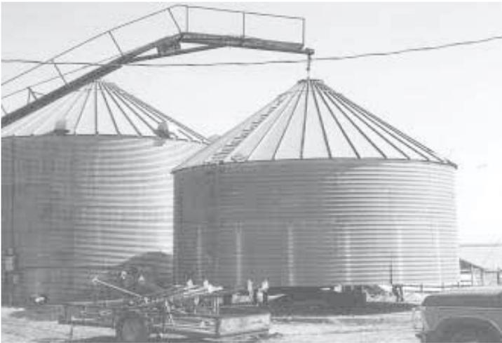
Pull-type boom is shown lifting top half of 10,000-bu. bin that Van Boening moved to another location.
