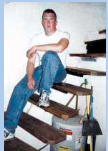
Furnace and water heater are hidden beneath a circular stairway that leads to top of silo.
