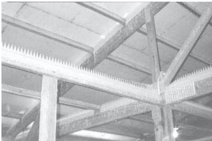
**“Birdblox”** anti-nesting and anti-perching strips snap onto top of 2-in. boards or rafters.
