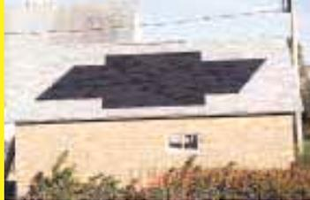
I started by making a shingle pattern graph on a piece of paper, and then drawing the bow tie to scale on the graph. The next step was to center the pattern on the room as best as possible. I spray-painted the design on the old shingles before tearing them off, and then counted the number of tabs between color changes.
