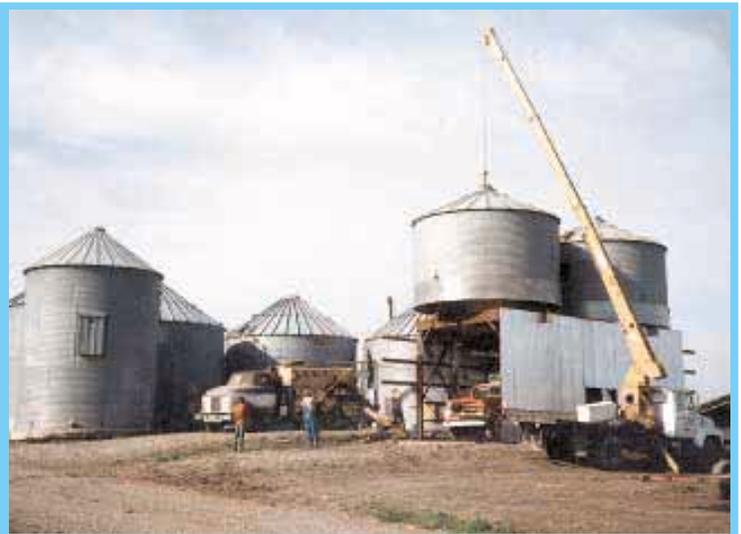
A crane operator was hired to lift bins on top of drive-through frame, which measures 16 ft. wide, 14 ft. high, and 36 ft. long.
