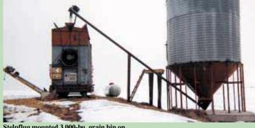
Stelpflug mounted 3,000-bu. grain bin on top of a home-built, 10-ft. tall steel hopper to make his own 4,000-bu. wet holding bin. Bin stands next to his continuous flow dryer (above). He made the hopper bottom out of 1/4-in. thick steel plate and mounted it on 16 steel legs that are anchored on 5-ft. deep footings (right).
