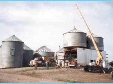
A crane operator was hired to lift bins on top of drive-through frame, which measures 16 ft. wide, 14 ft. high, and 36 ft. long.
