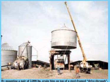
By mounting a pair of 2,000-bu. grain bins on top of a steel-framed "drive-through", Davies is able to load trucks fast.
