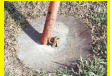
at one time or another. I set up a swing set for my three granddaughters and it didn't take long for it to start digging into the soft ground. This loosened the anchor rods and allowed the whole framework to sway back and forth. If left unchecked, the moisture in the ground would have corroded the legs.
