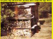
this idea. I got six metal crates from a local motorcycle shop for free. The crates are used to ship motorcycles. They give them away for free. I put some tin on top of the crates using self-tapping screws. I made a double layer of crates. It works great and keeps the wood real dry. (Glen Ray Goodson, 2205 Fairview Rd., Galax, Va. 24333 ph 540 236-3369)
