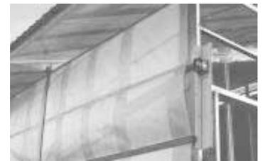
**"Sidewinder" curtain is designed to roll up tightly to the center. The top or bottom - or both - can be opened a little or a lot, depending on amount of ventilation needed.**
