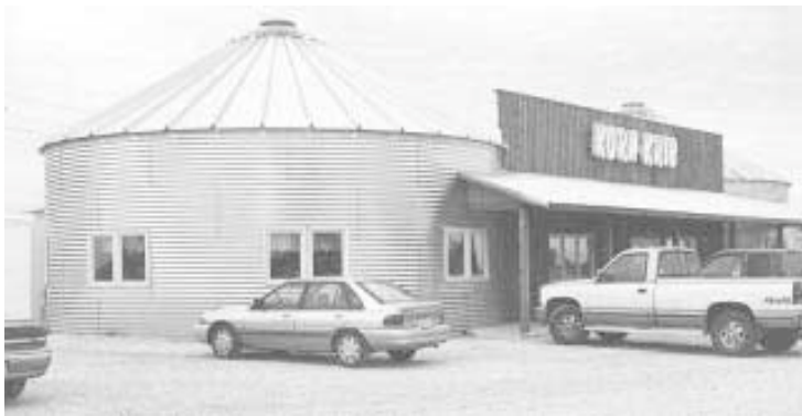
The new "Korn Krib", built out of a pair of grain bins, seats 175.
