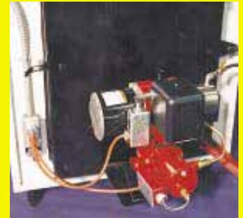
**Furnace burner uses a small 1/4-in. dia. piston to pump oil. A vein pump injects air into burner unit.**
