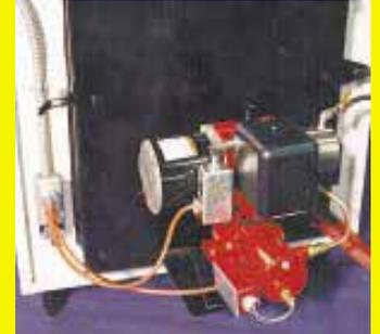
**Furnace burner uses a small 1/4-in. dia. piston to pump oil. A vein pump injects air into burner unit.**
