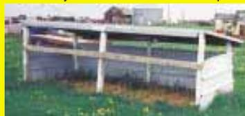
driven into the ground. I used four 10 ft. 2 by 4's for side, end and ceiling supports. Metal garage sections are screwed to the posts and 2 by 4's. I installed a couple old barn doors on top for a roof.
