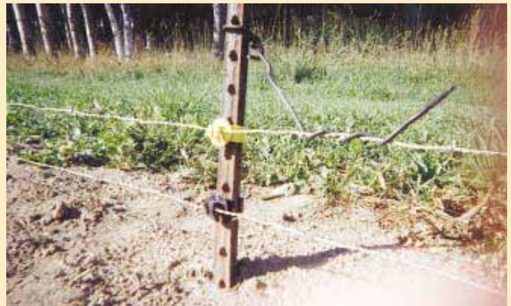
Two strands of light gauge electric wire run at 5 and 10 in. off the ground.
