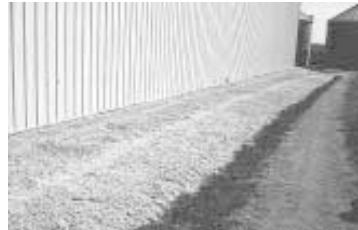
A 2-in. layer of loose rocks, laid on top of a layer of plastic, stops rodents from tunneling into building.
