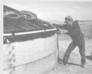
Curtis Hemstad bolts sheets of plywood together into a full circle and uses plastic to cover the grain.
