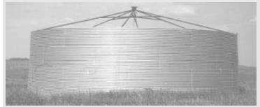
Jim Noram's temporary grain bin has no permanent roof or floor, which saves greatly on cost.
