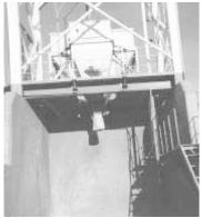
The tank stands on four legs fitted with weigh scales so cement and sand can be weighed as it's dumped into a mixing truck.
