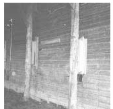
Five poles were set along the outside wall. Threaded redi rod was used to draw the walls to the poles.
