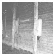
Five poles were set along the outside wall. Threaded redi rod was used to draw the walls to the poles.
