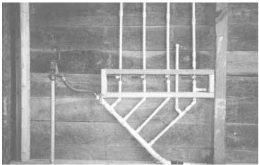
This plumbing setup in McCarthy's barn makes it easy to drain pipes in freezing weather.
