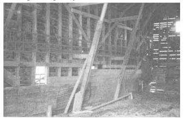
Poles were set in the ground inside to brace walls and roof.
