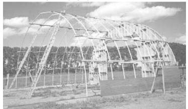
Lightweight tubing, commonly used in oil fields, was used for the framework.
