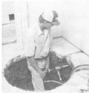
The first step is digging a 42-in. dia. hole in basement floor (left). Then lateral lines are drilled under the floor using a patented process (right).
