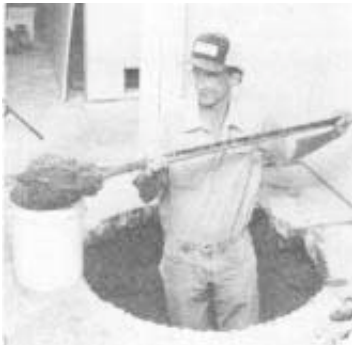
The first step is digging a 42-in. dia. hole in basement floor (left). Then lateral lines are drilled under the floor using a patented process (right).
