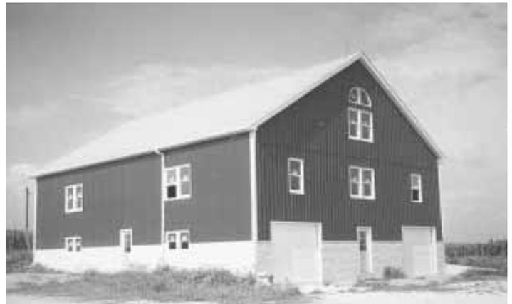
The barn as it looks today. The crumbling old foundation was replaced with new concrete and the barn was sided and roofed with steel siding.
