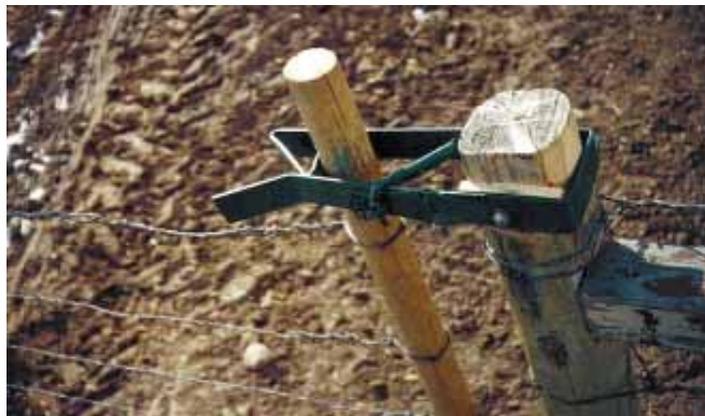
The latch is made from strap iron and bolts to both sides of a squared off fence post.
