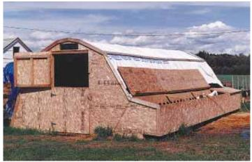
Borst spent only about \$600 to build this 14-ft. wide, 30-ft. long, and 9-ft. high "hoop-type" building that has a roof made out of plastic silage bags.
