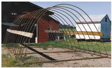
Building's arched framework is made from 25-ft. lengths of sucker rod and 7/8-in. dia. drill stem pipe. The rods are secured to a rectangular frame welded together from 2 5/8-in. dia. drill stem pipe. To make arch more uniform and rigid he fastened a pair of wooden boards to rods along each side of the arch about 4 ft. off the ground.
