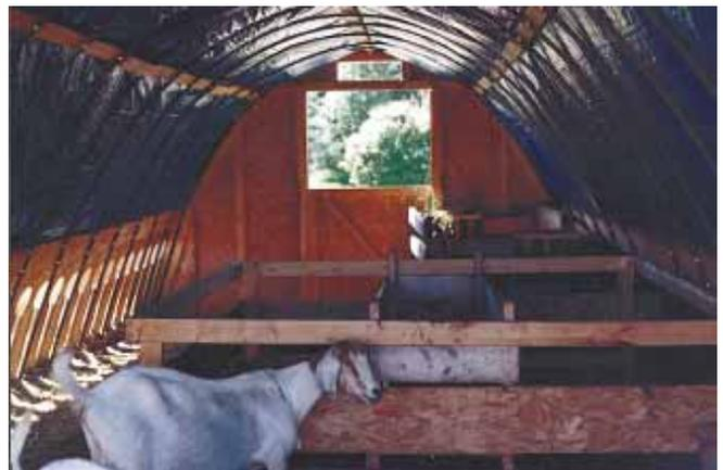
Borst built an 8-ft. sq. creep feeder inside building. To make the feed bunk alongside the building, he cut a series of 8-in. dia. holes in plywood spaced every 2 ft.
