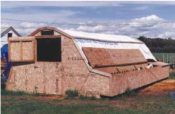
Borst spent only about \$600 to build this 14-ft. wide, 30-ft. long, and 9-ft. high “hoop-type” building that has a roof made out of plastic silage bags.
