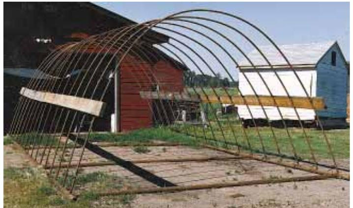
Building’s arched framework is made from 25-ft. lengths of sucker rod and 7/8-in. dia. drill stem pipe. The rods are secured to a rectangular frame welded together from 2 5/8-in. dia. drill stem pipe. To make arch more uniform and rigid he fastened a pair of wooden boards to rods along each side of the arch about 4 ft. off the ground.
