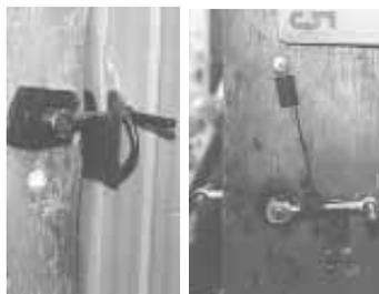
Long-lasting "bike pedal" latch fits in existing lock hole in door.
