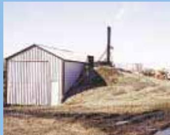
Furnace is buried in an earth berm next to a 16 by 32-ft. shed. The Klimacks burn about 40 5 by 6-ft. round bales of flax straw a month in the coldest weather.
