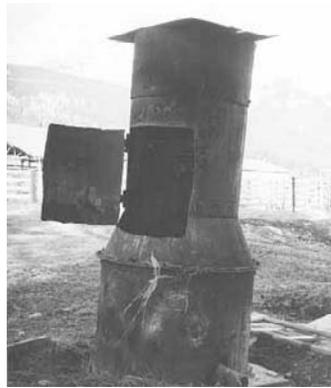
Incinerator consists of a 6-ft. dia. barrel with a 4-ft. dia. barrel mounted on top.
