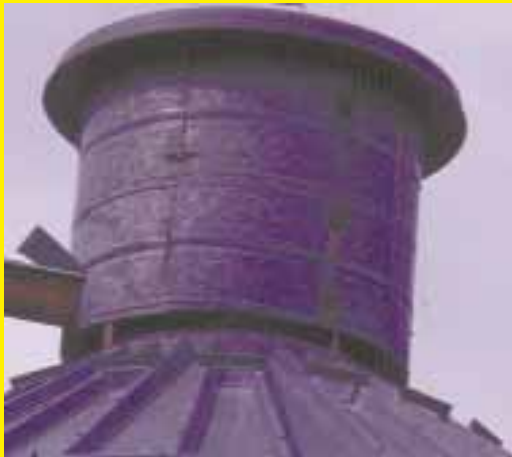
Young used the top two sections of an old round hog feeder to cover bin opening.
