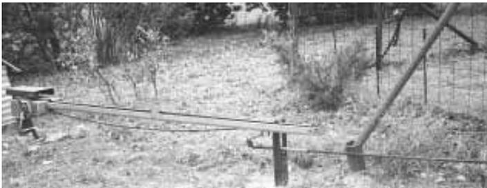
Gate opener built from a conventional garage door opener is used to open and close a 16-ft. steel gate across Wilson's driveway.
