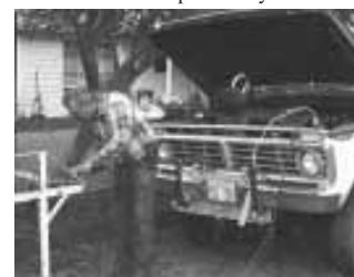
Premier Power Welder that mounts underneath the hood of a pickup (Vol. 19, No. 4),
