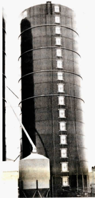
Company converts Harvestores to top unloading for less than the cost of a rebuilt bottom unloader (see other pictures on p. 1).
