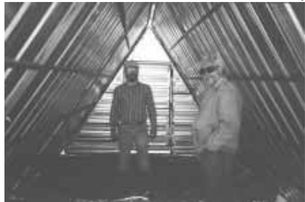
Each panel is braced with three 1-in. sq. tubing cross members.
