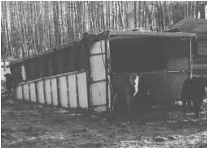
Shelter was made by turning two gravel truck boxes upside down and mounting them at an upward angle on skids. Open end is 6 ft. high; back end 3 1/2 ft. high.
