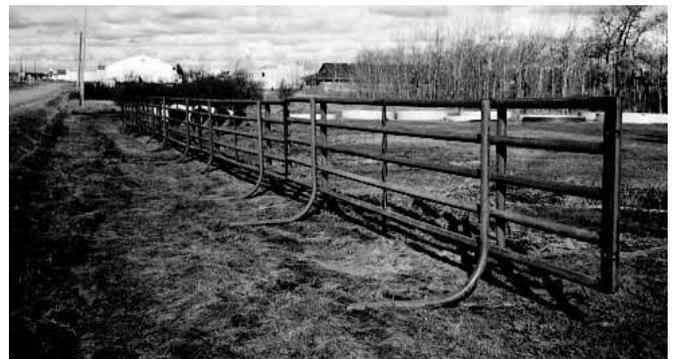
Self-supporting fence panels are equipped with a pair of steel legs on each side that eliminate need for posts and allow panels to be easily moved around.
