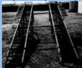
Ramps are 3-in. channel iron and 1 1/2-in. angle iron, with plywood catwalks.
