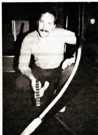
Each 9-in. Shin Guard strip is serrated in 1-in. increments.
