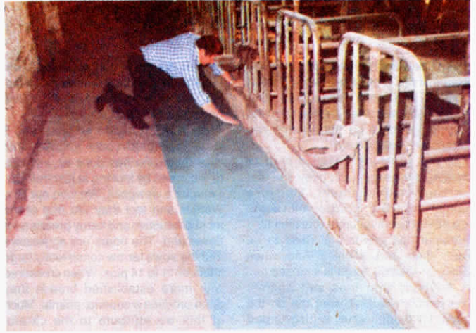
Epoxy's also applied to manger and feedbunks because it's smoother on a cow's tongue than rough concrete.
