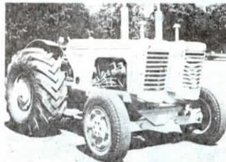
32 years ago Oliver came out with a commercial "Siamese Twin" tractor that used two industrial 880 tractors with single front and rear axles but with dual transmissions. I saw this tractor in Lincoln, Neb., at a field day in 1960.
