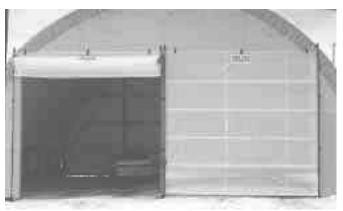
Winch-operated canvas end doors roll up or down on a track like a garage door and seal tight against building so they won't flap around in the wind. (Canadian); a kit for a 15-ft. high door sells Conrad Klassen, Box 389, Altona,
