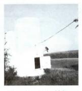
"Pieces of 6-in. dia. pipe, 2 ft. long, are used to make auger openings near the bottom of the tank. Ladders are made by bending 5/8-in. dia. round stock into square 'U-bolts' that are placed in holes in bin wall and then welded in place. A piece of 5/8-in. flat stock is welded across inside of tank where steps are affixed.
