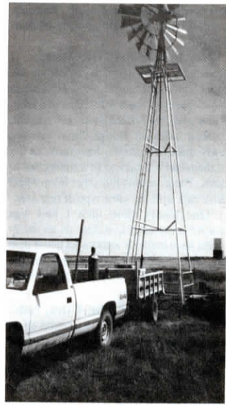
To drop windmill to the ground, Carroll releases the locking hinges and jacks up one side, lowering it to the ground with a cable hooked to a pickup.
