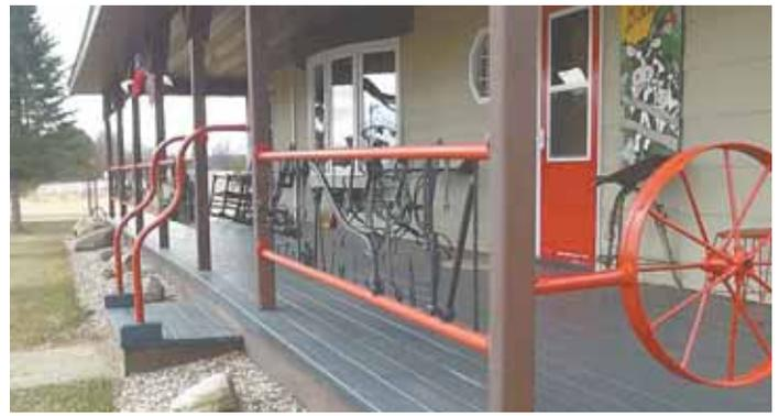
Ron arranged the wrenches between sections of steel pipe and welded them in place. Then he spray painted the railings black.
