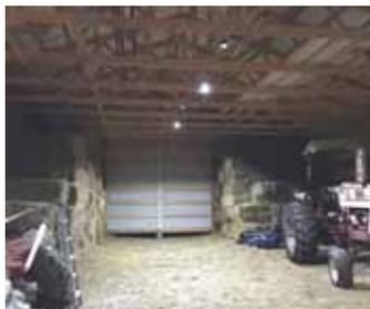
Dennis Gilliland connected a 3 1/2-watt solar panel to a deep cycle marine battery, allowing him to energize four 10-watt LED portable work lights in his barn. Panel mounts on homemade brackets outside barn.
