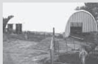
Roger Zummach put up this wood hoop livestock building with two doors on one side and a single door at one end. It measures 36 by 90 ft. and is 18 ft. high.
