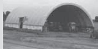
This shed with steel trusses measures 50 by 112 ft., with a 27-ft. high center. He keeps machinery in one half of the building and hay and straw in the other half.
