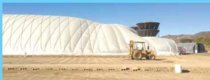
Airflow is produced by two 20-ft. dia. towers at one end of greenhouse. Four high-speed fans suspended in each tower keep air pressure constant.
