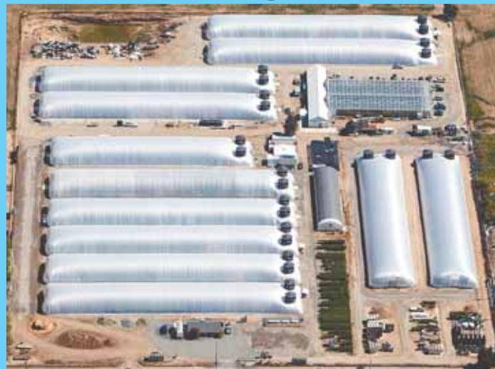
Airstream Innovations greenhouse tunnels are helping plants grow faster at BZ nursery due to the 3 mph flow of air across the plants. Pressurized air also keeps each tunnel's 66 by 360-ft. plastic roof inflated.
