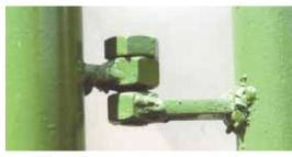
A simple nut-bolt combination can be used to make a sturdy gate hinge.
